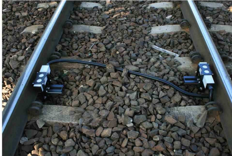
Fig. 2. Two measurement antennas mounted to the rails
